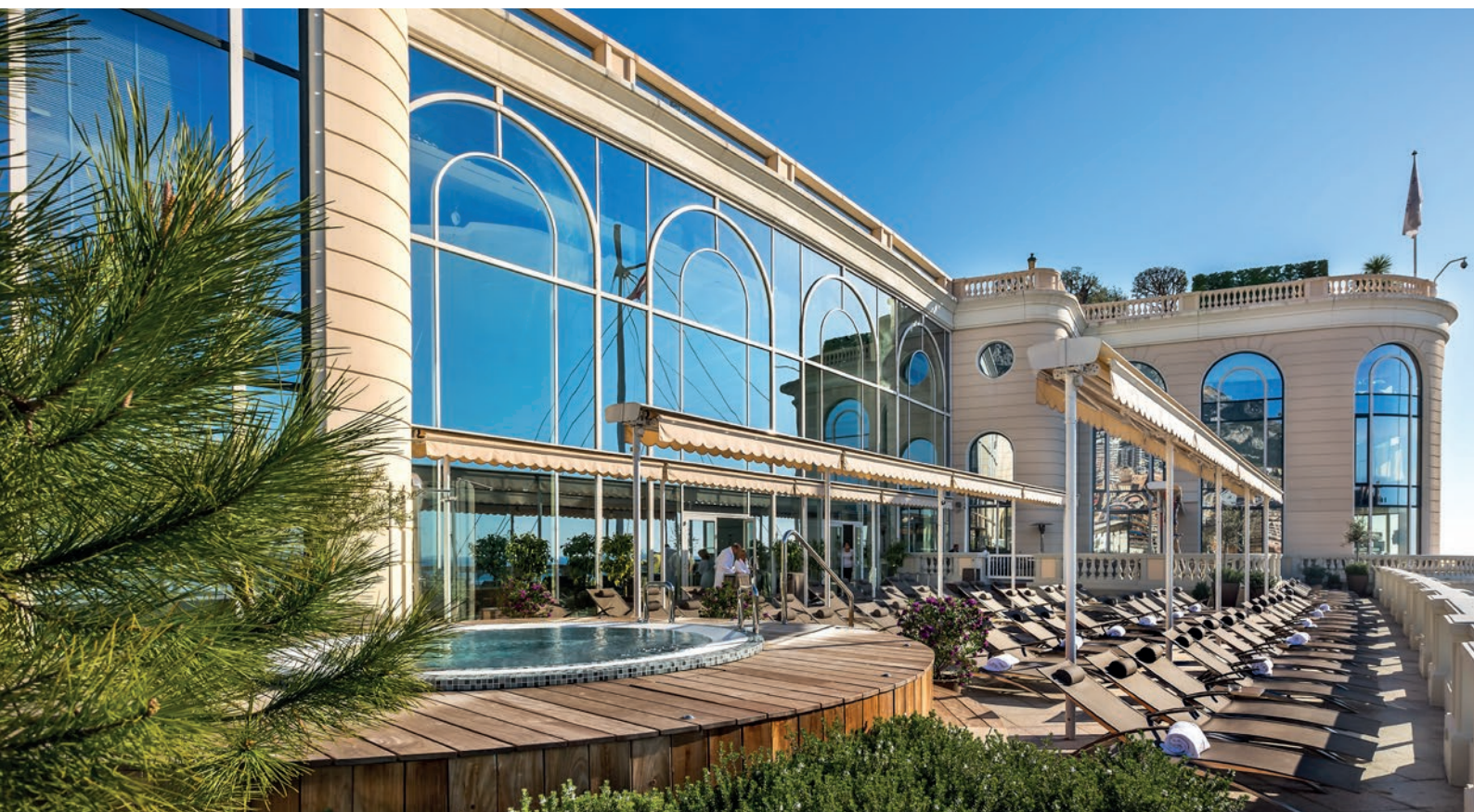
MONTECARLO THERMES MARINS SBM_TH-Exterior-View
